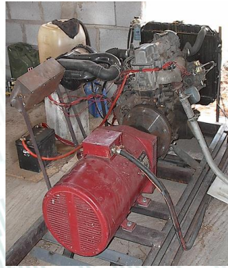
Engine with 20kVA generator
