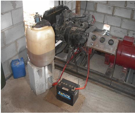
Engine with 20kVA generator
