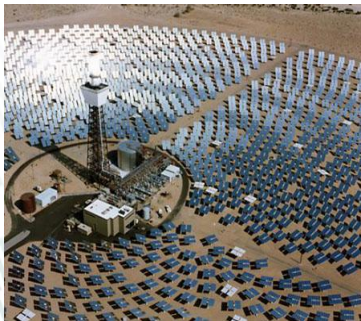
Solar tower in Barstow, California
